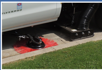
VACUUM AND BRUSH REMOVAL OF DEBRIS
